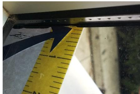
Figure 3.2.2, Primary Sealant in Sightline
