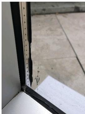
Figure 3.2.1, Primary Sealant in Sightline
