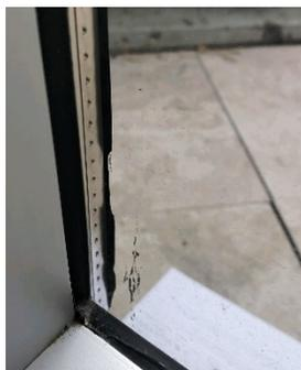
Figure 3.2.1, Primary Sealant in Sightline
