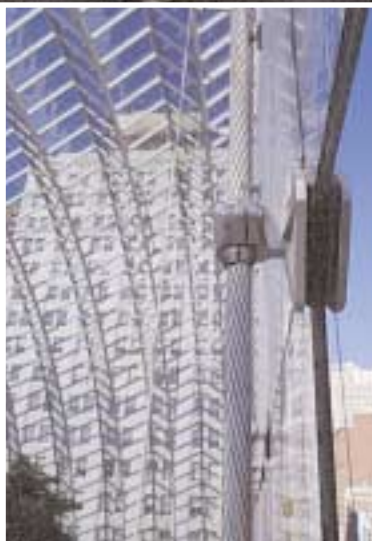
A cable net served as the backing system on the Kimmel Center.
