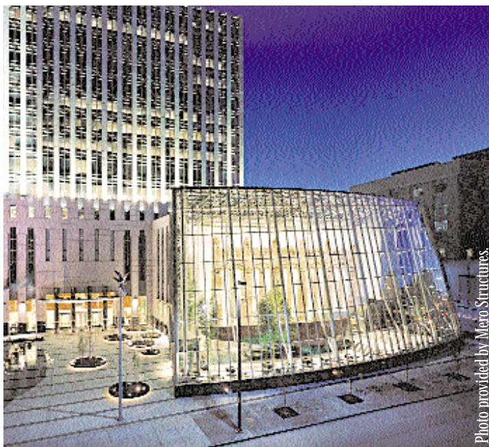
First National Center, Wintergarden, in Omaha, Neb., constructed by Mero, is an example of a point-supported glass facade.
