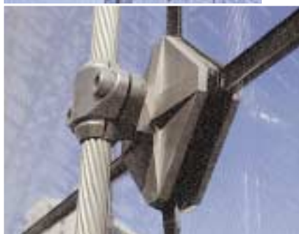
A cable net served as the backing system on the Kimmel Center.
