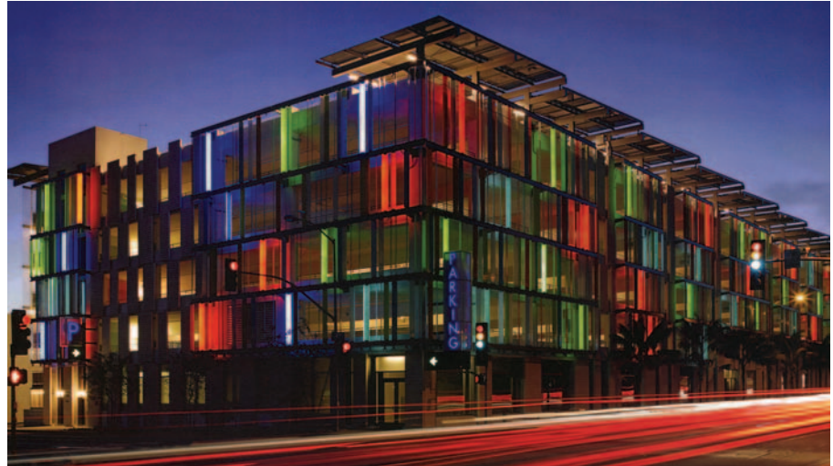
The Santa Monica Civic Center Parking Structure blended tempered and colorful laminated glass. It won the Tempered Glass—Commercial category.
