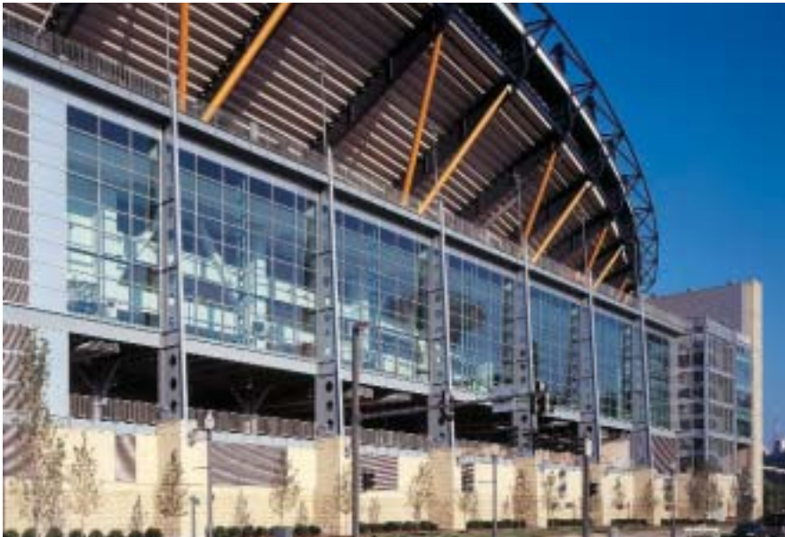
High performance glass products have allowed designers to expand glass in innovative applications for sports facilities, such as the glass curtainwall on Heinz Field in Pittsburgh, Pa.
